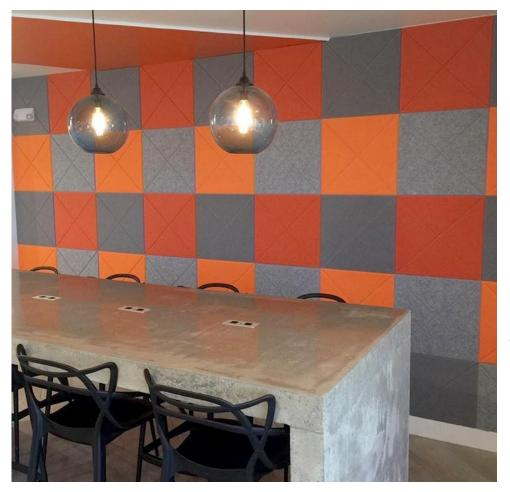
"Besides attenuating reverberation, these wall treatments mitigate annoying echoes off the back wall and flutter echoes. Sometimes diffusion panels or wall shaping can break up these echoes as well." These are basic fixes and are mostly recommended for spaces on a budget.
